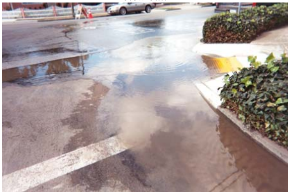
Saturday, February 26, 2011. Water pipe cap popped up 800 Blocks of Borregas and Carolina Avenues.
