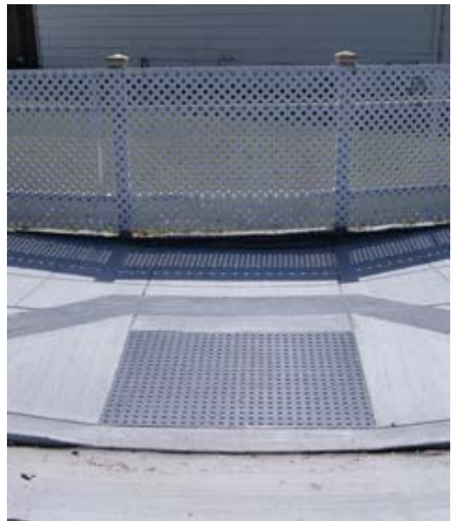
One of the new corner curbs on Duane and Kirk
