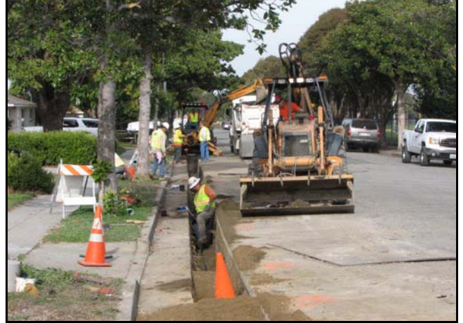
San Diego Avenue gets a new water main.
