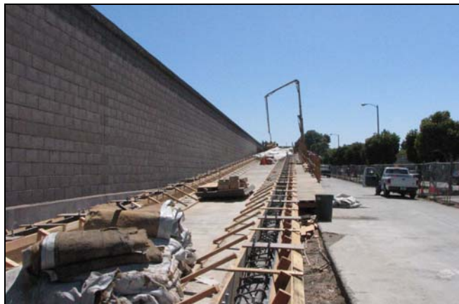
Pouring cement for the new bike bridge.
